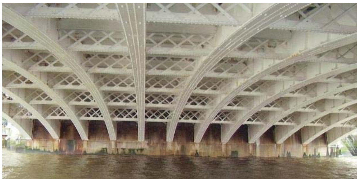
Figure 2. View of the underside of the bridge
