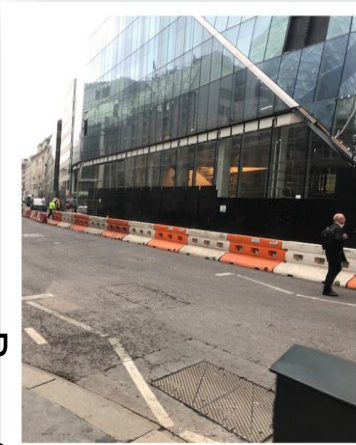
Road narrowed due to construction
