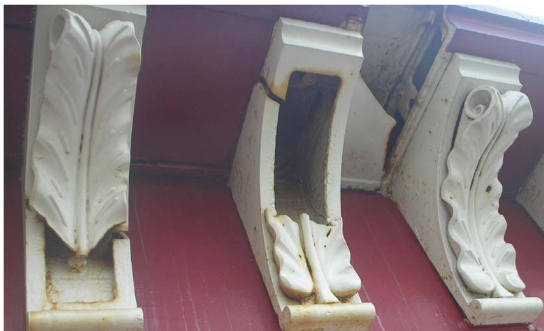
Figure 146. Current rust staining on the bridge
