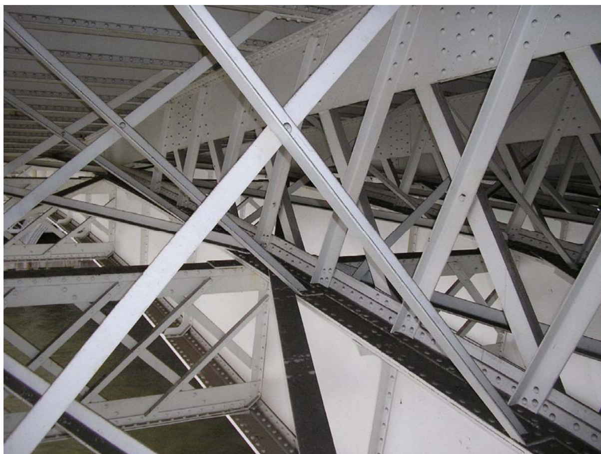
Figure 3. Braces between arch ribs
