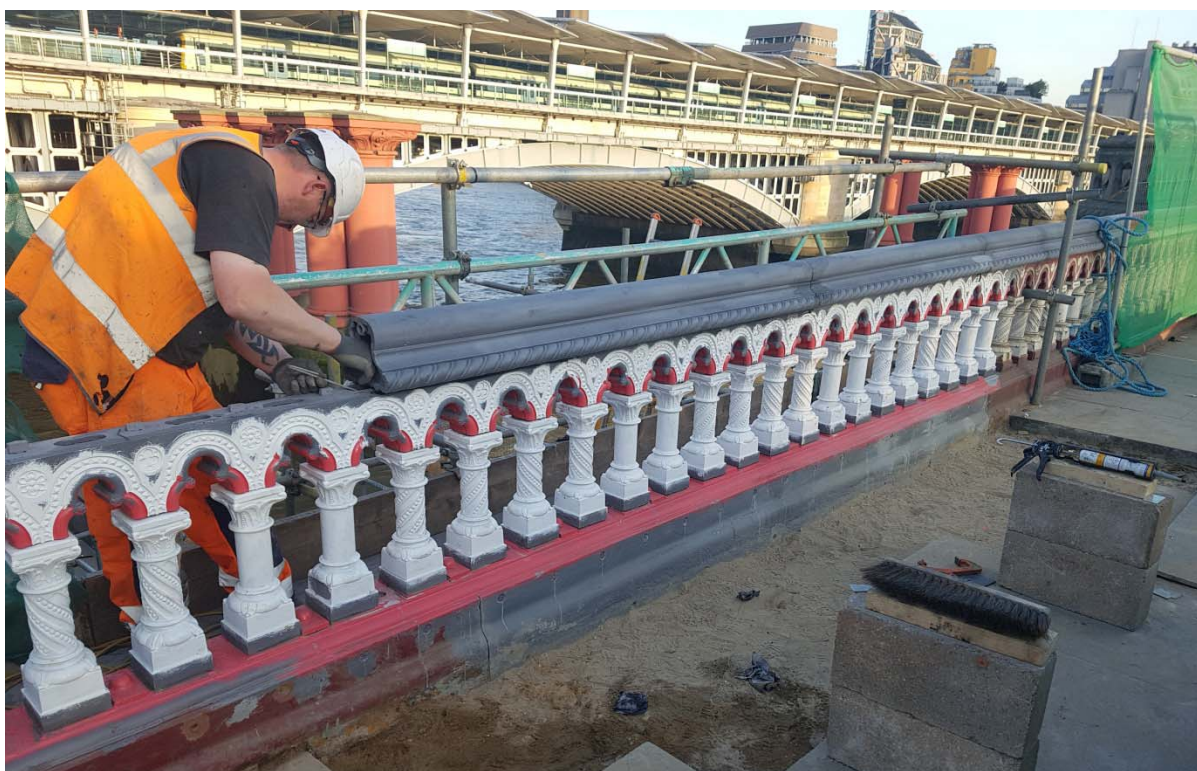
Figure 12. Parapet Reconstruction
