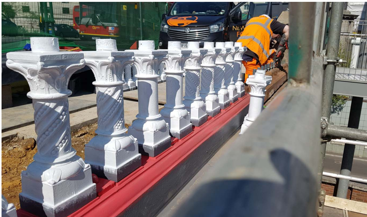
Figure 111. Parapet Repairs
